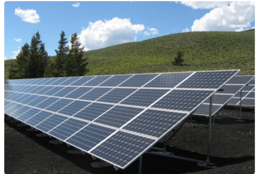
Solar Panels on a hill side
